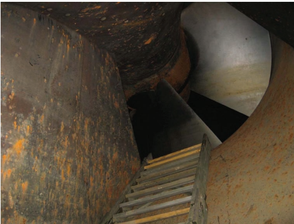
Photograph 5: Turbine Runner Blades
