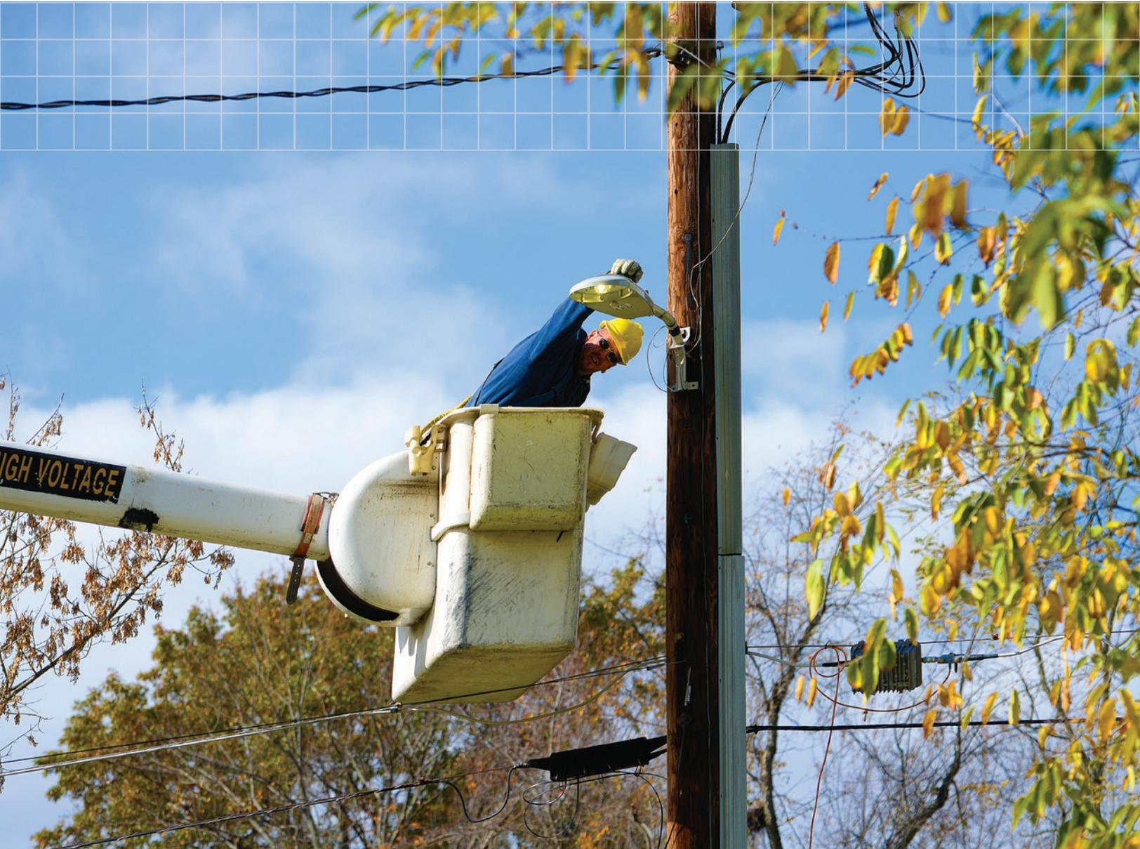
*Several participating AMP member communities have upgraded to higher-efficiency street lighting through the Efficiency Smart program, which provides rebates on top of the cost savings from reduced power use. Shown here is a Georgetown Electric Department crew working on an LED street lighting project completed in 2014.*
