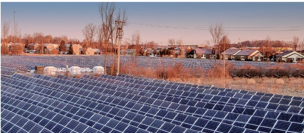
*AMP developed and managed construction of the 3.54-MW (AC) Napoleon Solar Facility (shown here), which was completed in 2012 and is connected to the electric system of AMP member Napoleon. AMP continues to pursue solar and natural-gas options for behind-the-meter generation in its member communities.*
