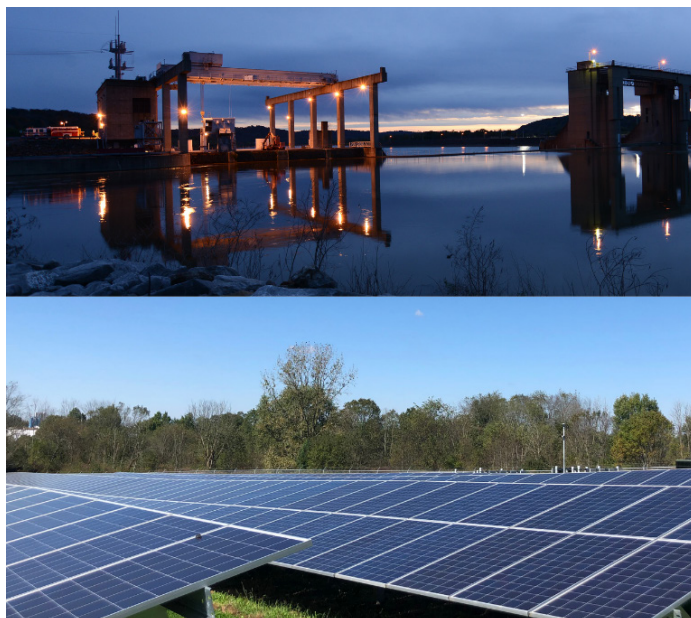
The Bellevalle Hydroelectric Plant (top) and Brewster Solar Field (bottom)
