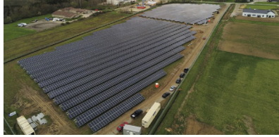
The final Solar Phase II site in Wadsworth
